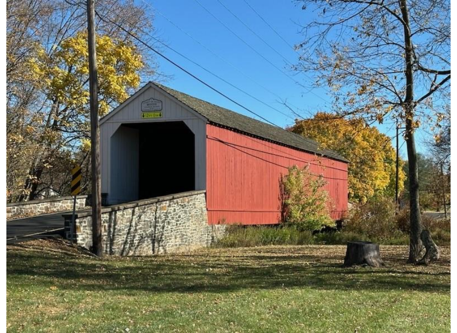
Pine Valley Covered Bridge – built in 1842
